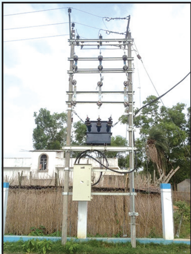
DTR with Strutcure installation – Mukundapur CCC, Kandi, Murshidabad District
